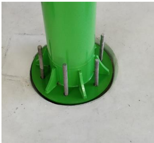
Figure 2: Baseplate with Pad Leveling
