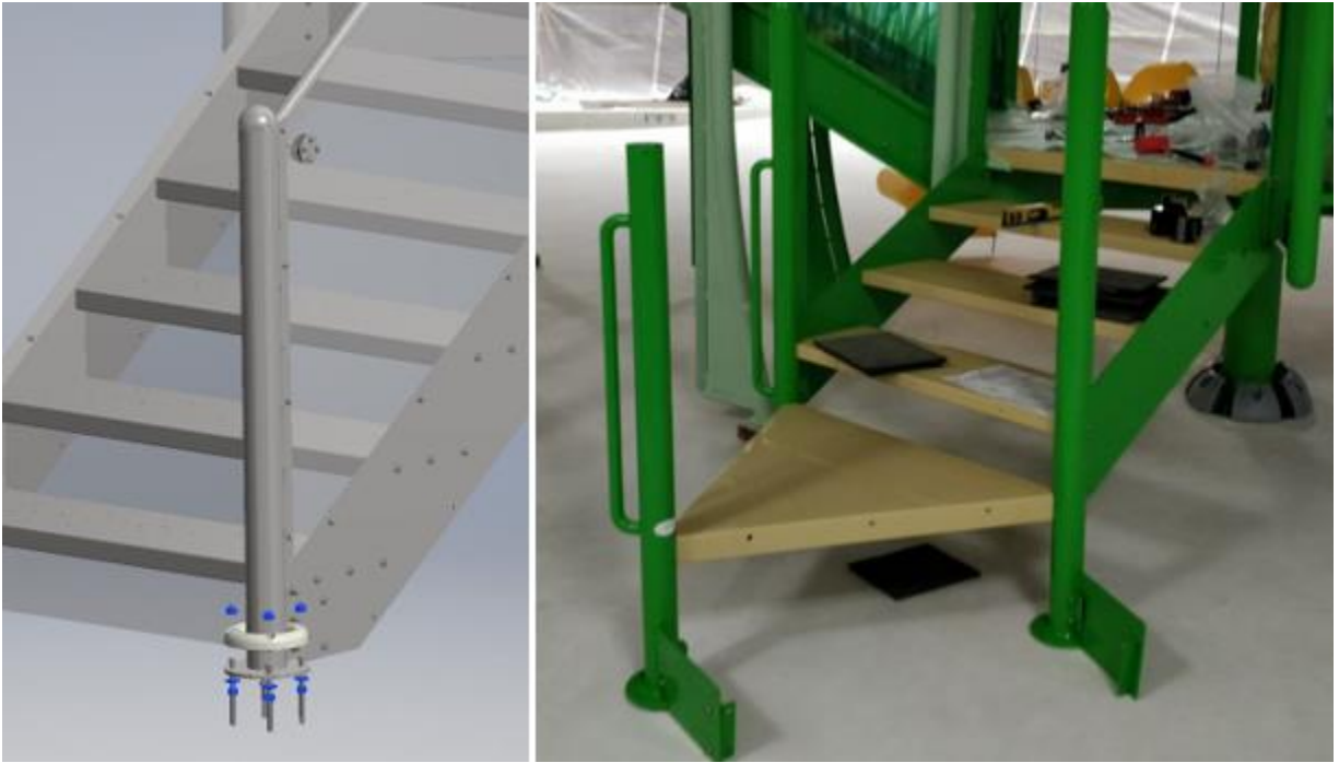
Figure 16: Stair Column Assembly
