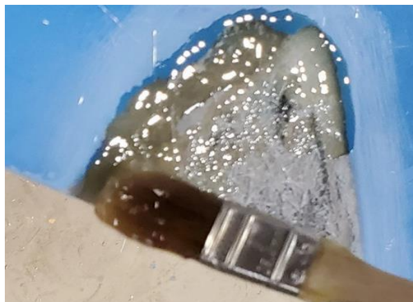
Figure 35: Wet Repair Area with Resin Mixture
