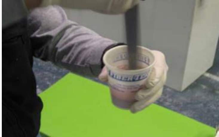
Figure 49: Mix Gelcoat and Pro Patch
