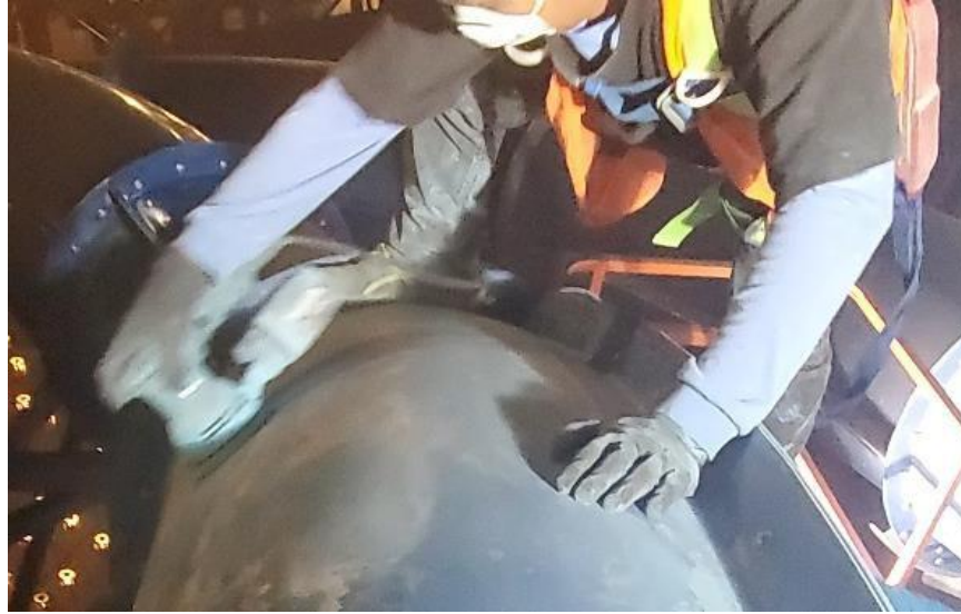
Figure 70: Sanding FRP for Clear Coat
