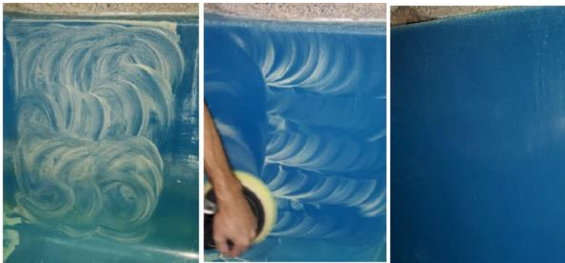
Figure 6: Buffing and Waxing Shutdown Lane FRP
