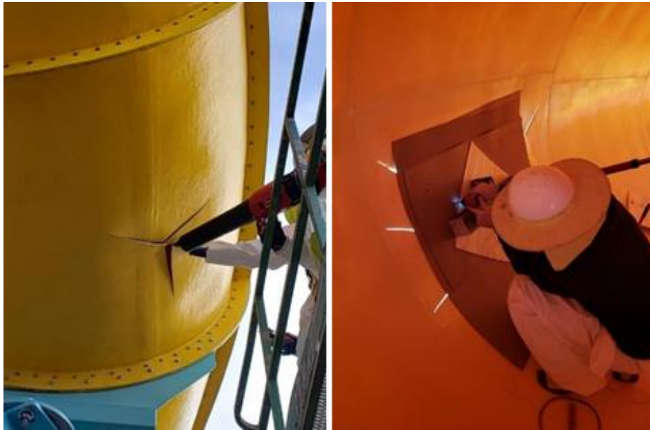
Figure 62: FRP Deformation Repair Preparation
