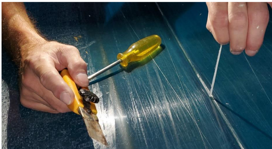
Figure 7: Removing Old Filler
