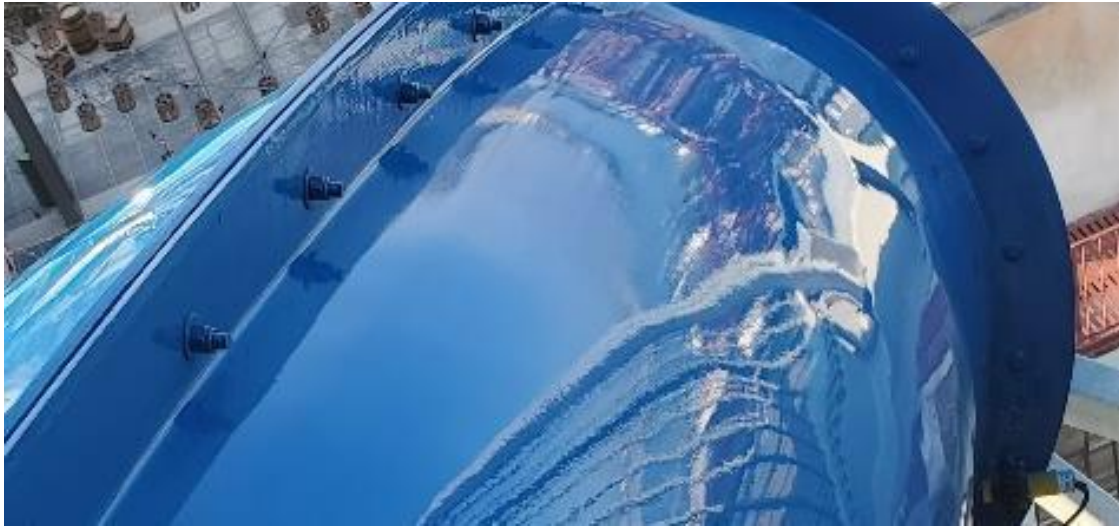
Figure 73: Inspect Finished FRP for Drips or Runs
