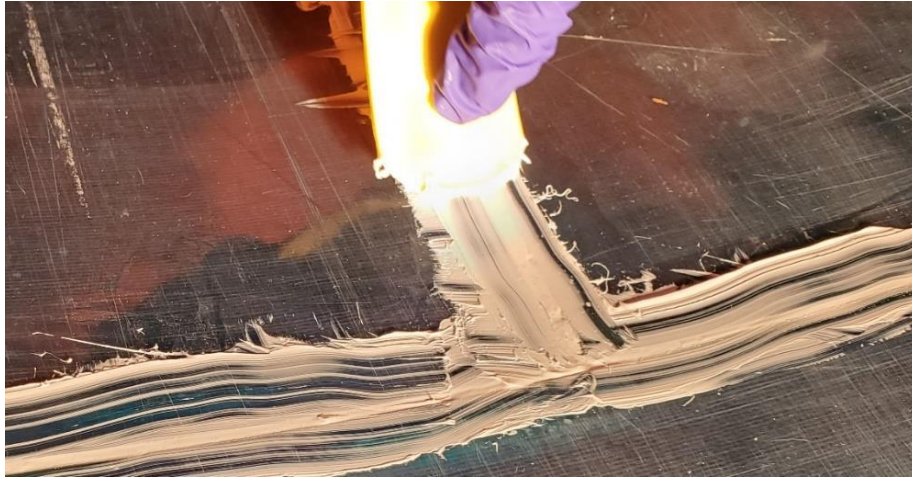
Figure 12: Press in New Filler
