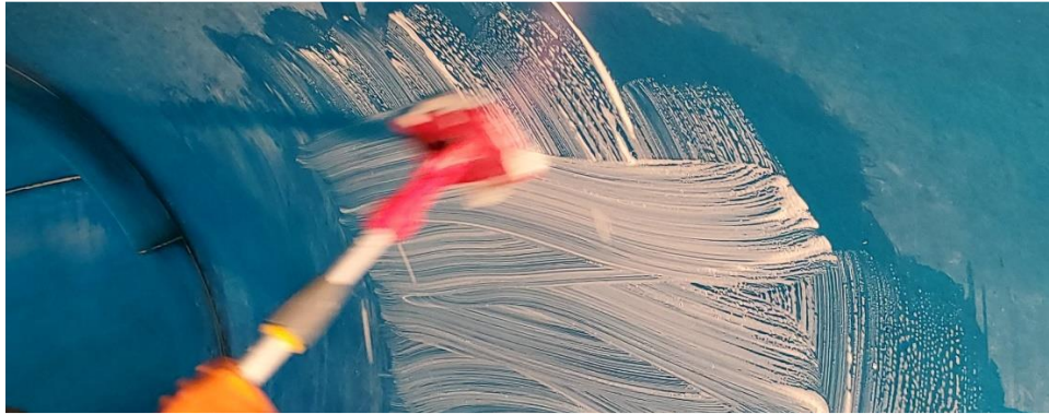
Figure 5: Scrubbing Calcium, Lime, and Rust Remover on FRP
