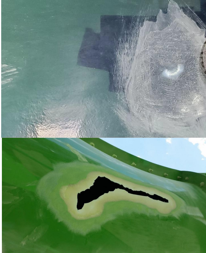
Figure 30: Grind and Sand Edges of Repair Area
