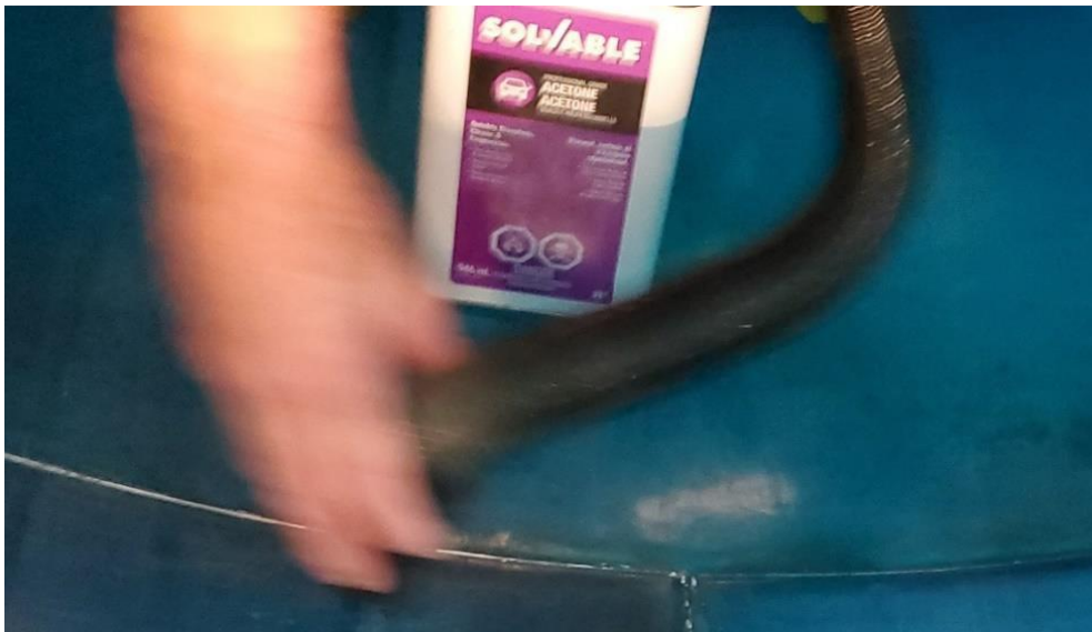
Figure 9: Vacuum and Clean Joints with Acetone
