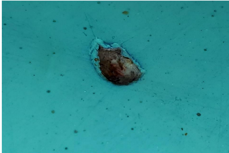
Figure 20: Small Chips in FRP
