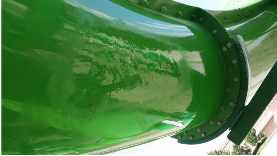
Figure 56: Gelcoated Large Repair, Outside
