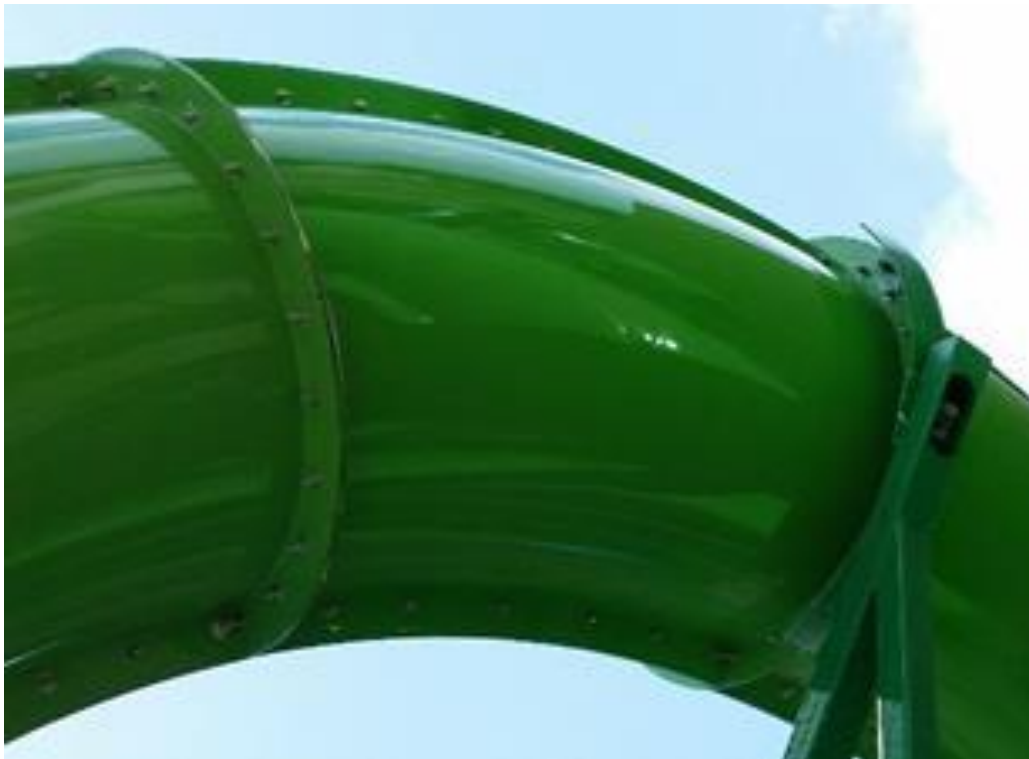
Figure 74: Buffed and Clear Coated Large Repair, Outside
