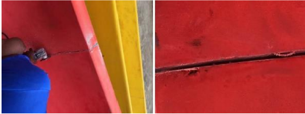
Figure 8: Mechanically Remove Filler and Deburr Edges
