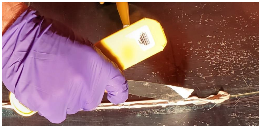
Figure 11: Pack in Joint Filler
