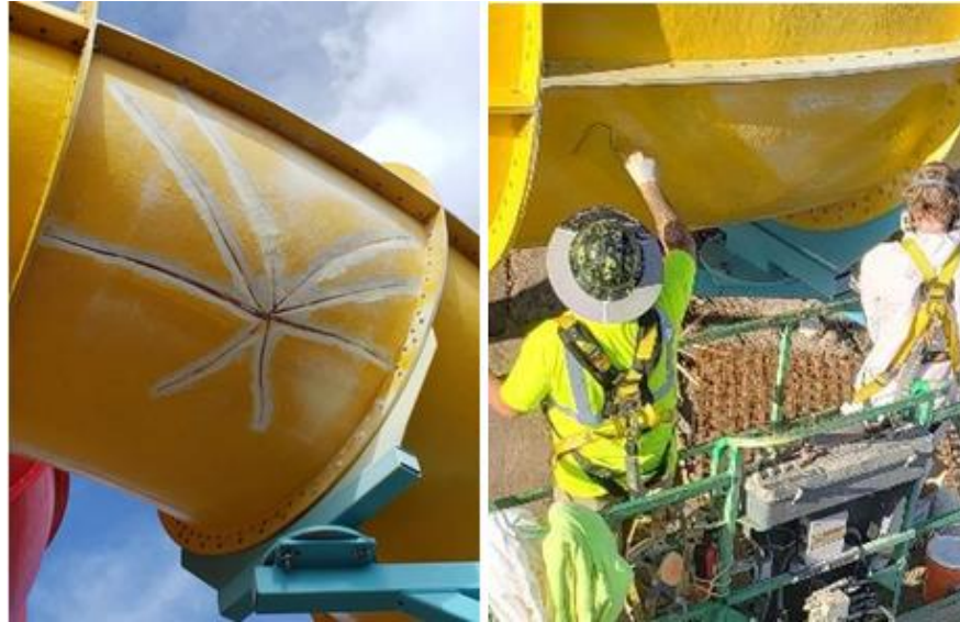
Figure 63: FRP Deformation Repair Grinding and Fiberglass Application
