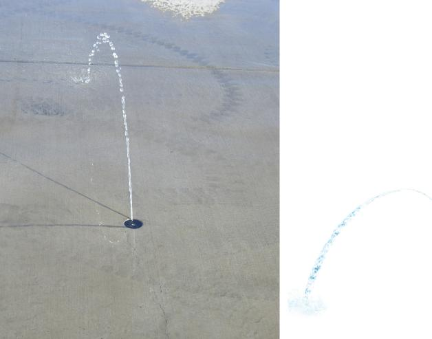
This adjustable ground spray shoots a single arching stream of water. Using a tool, the ball in the nozzle can be easily adjusted to shoot the stream in another direction and water pressure can be adjusted to affect height and reach. Kids of all ages will want to reach out and touch this steady stream of water.
